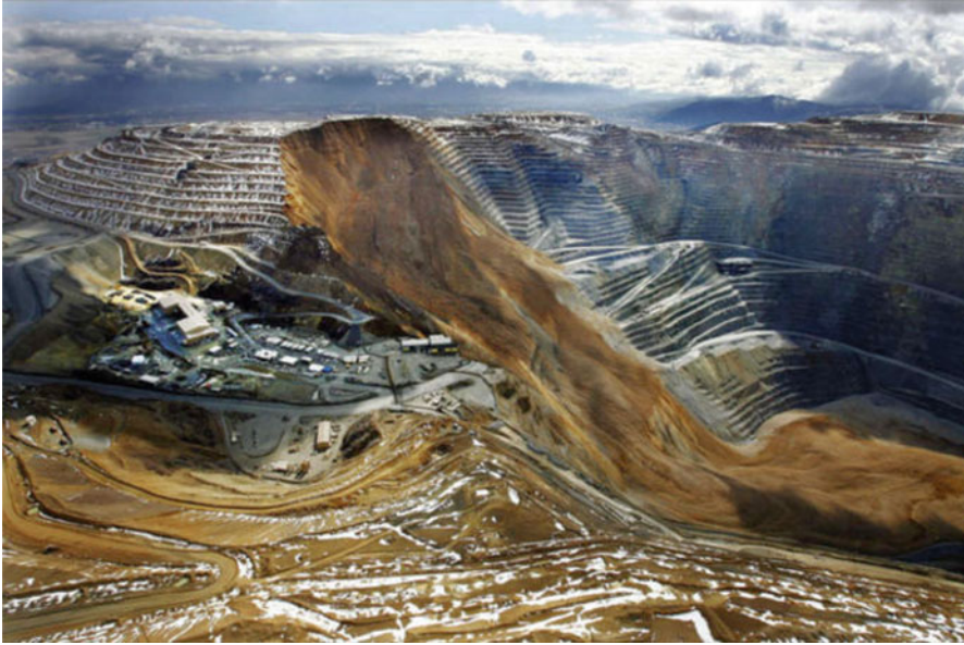
Fig. 4 Slope failure in Bingham Canyon mine [58]
